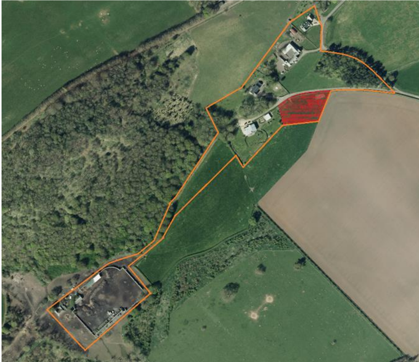
Fig 4: Annotated aerial image of existing Building Group at the former Stichill House with application site in red wash and natural boundaries illustrated (in orange).
